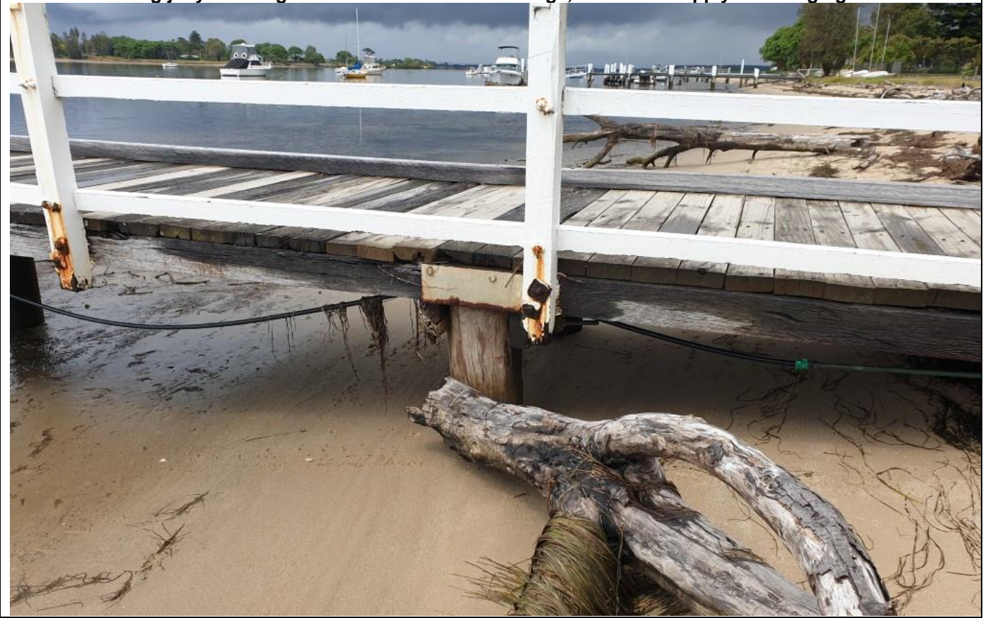
Photo 5. Existing jetty showing deteriorated timber and fixings, and water supply line hanging below
