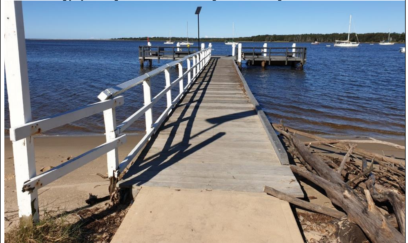
Photo 3. Existing jetty showing deteriorated timber railing and rusted fittings
